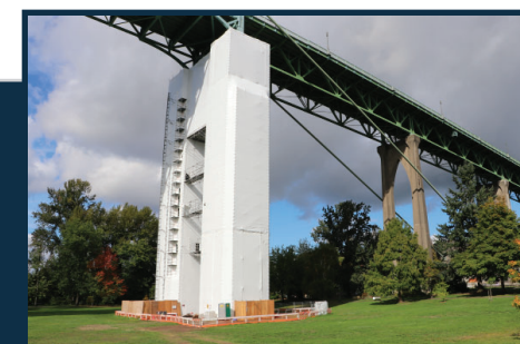
A column wrapped during construction under the St. Johns Bridge.
