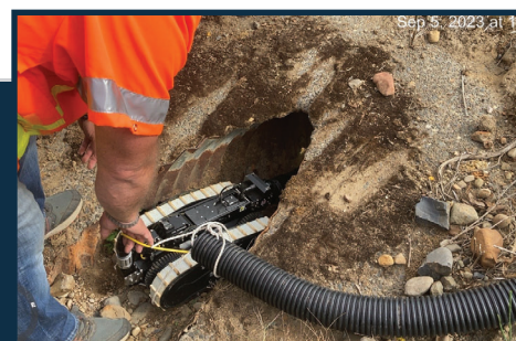
Crews guide camera into culvert to assess conditions.
