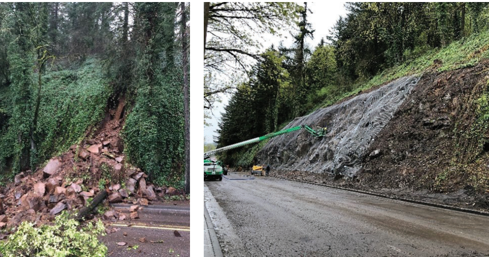
Above: At left, the January 2022 landslide at NW Bridge Avenue (U.S. 30 Bypass). At right, crews drill the last of the anchors in the pinned mesh system, April 20, 2022.
